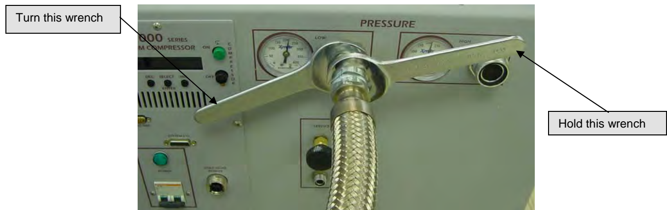
Figure 7-1: Disconnecting flex lines from a compressor package
